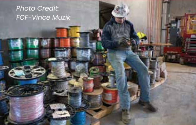
Beltrami Jail – Ryan Sharp, a pipefitter for UA Local 11, sits on a stack of wires at the construction site of Beltrami County’s new Adult Corrections Center in Bemidji, MN. The target date for completion is March 2027.
