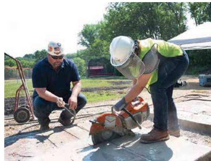
Alli Westra-Smith of New Country School in Henderson, Minn., saws through concrete as Stacey Karels of Laborers Local 563 sprays water.
