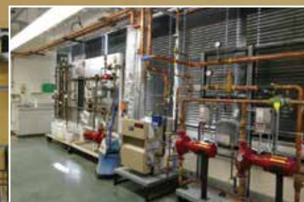
The Sheet Metal Workers Local #10 JATC Credit: FCF Staff
